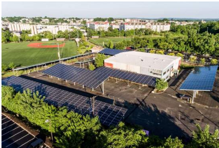
Image 10. Solar carport installation. Photo credit: Ecogy Energy.
