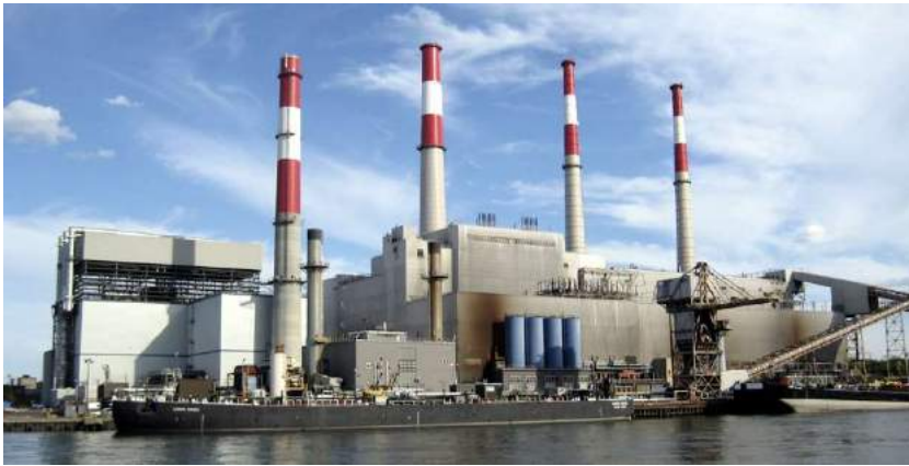
Image 3. Ravenswood Generating Station, Long Island City, Queens. Photo credit: Wally Gobetz, 2007.
