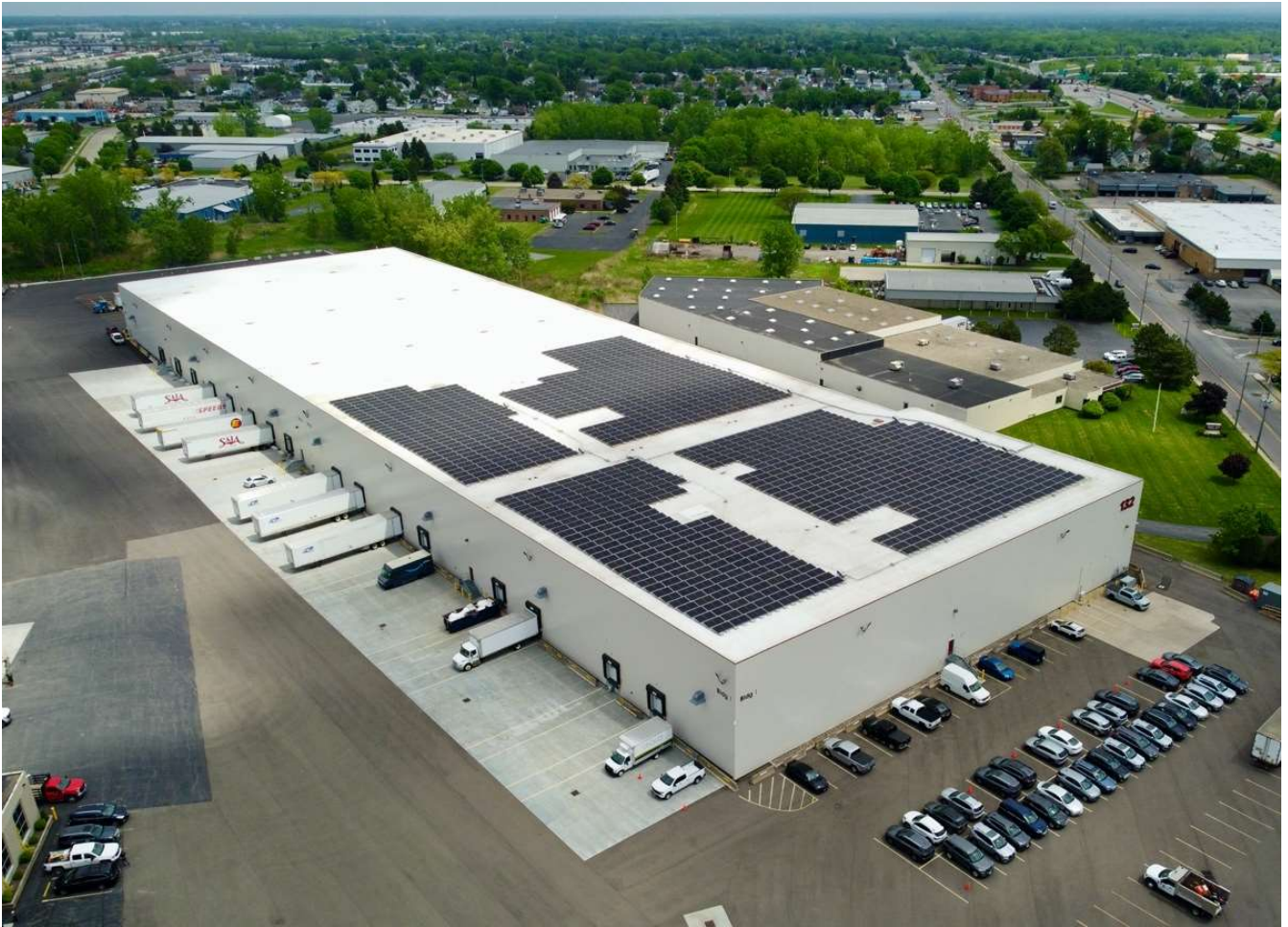
Image 11. Commercial rooftop solar installation in Buffalo, NY. Photo credit: Pinto Construction Services, Montante Solar.
