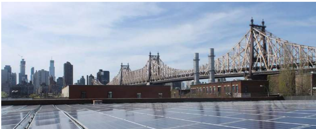
Image 1. Solar installation in front of Queensboro Bridge in New York City. Photo credit: NYSEDA.
