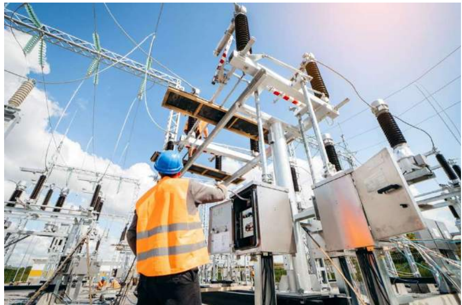
Image 15. Utility engineer inspecting substation electrical infrastructure. Photo credit: Sunco.
