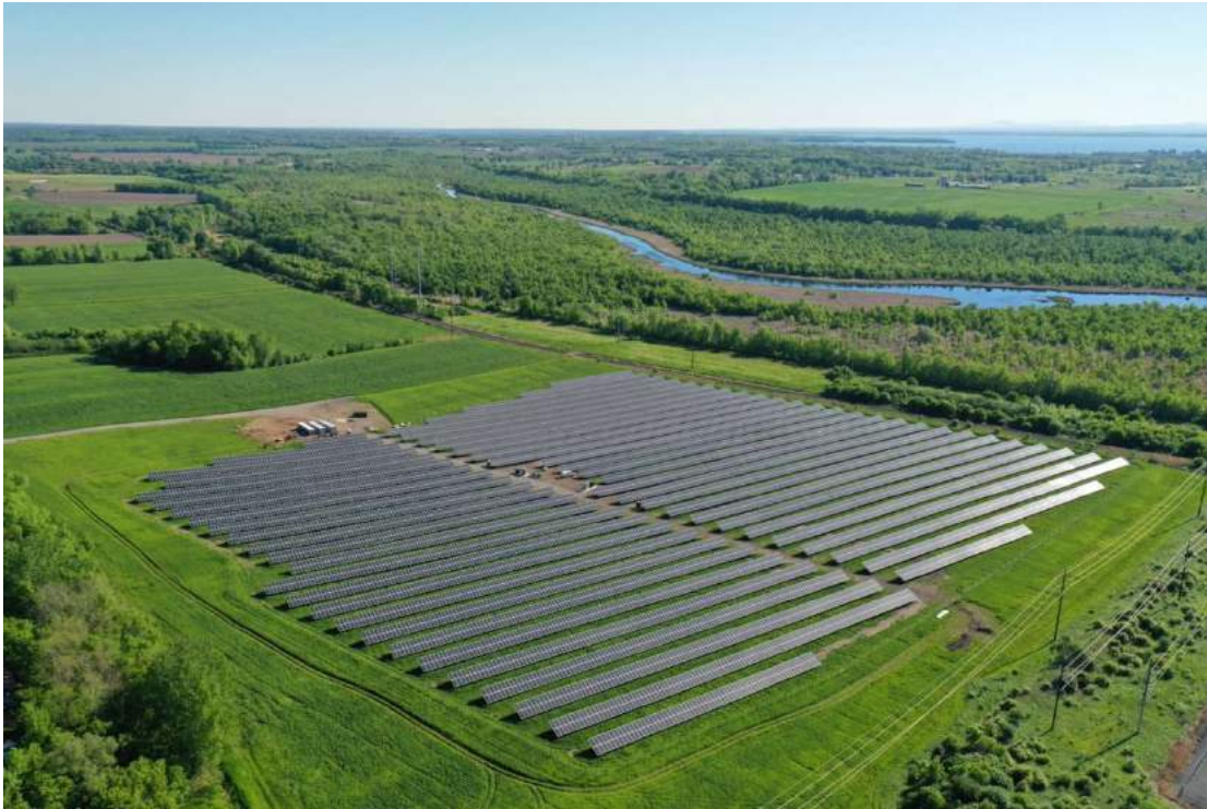
Image 6. Ground mount community solar array, Upstate New York. Photo credit: GreenSpark Solar.
