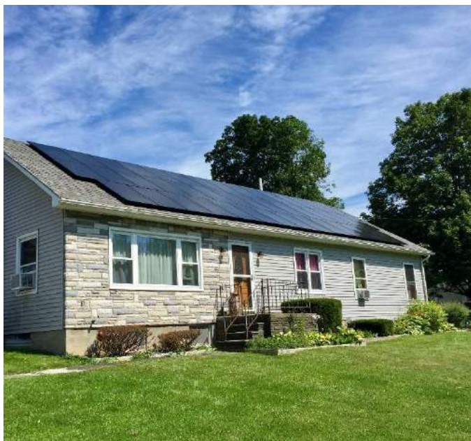
Image 16. Residential solar installation. Photo credit: Kasselman Solar.
